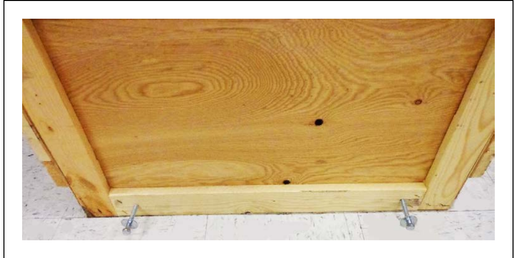
Figure 3-4. Crate Bottom-rear Lag Bolts
